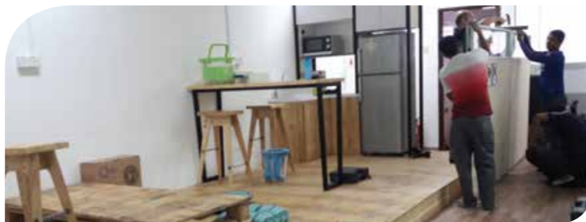
Eco Pantry under renovation.
