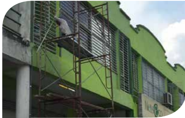
Paint work in process.
